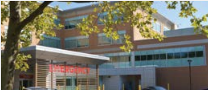
The UM Charles Regional Medical Center Emergency Department expansion and renovation project is complete with a larger, more comfortable waiting room and more handicapped and close-in parking.
