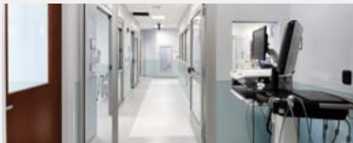
The new section of the Emergency Department houses patient rooms, including several dedicated to caring for behavioral health patients waiting for a transfer to another facility. It also features an enclosed nursing station and new patient bathrooms and showers.
